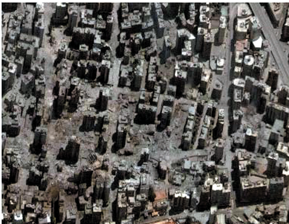
DAHIEH, LEBANON (AFTER) Photo taken July 22, 2006
